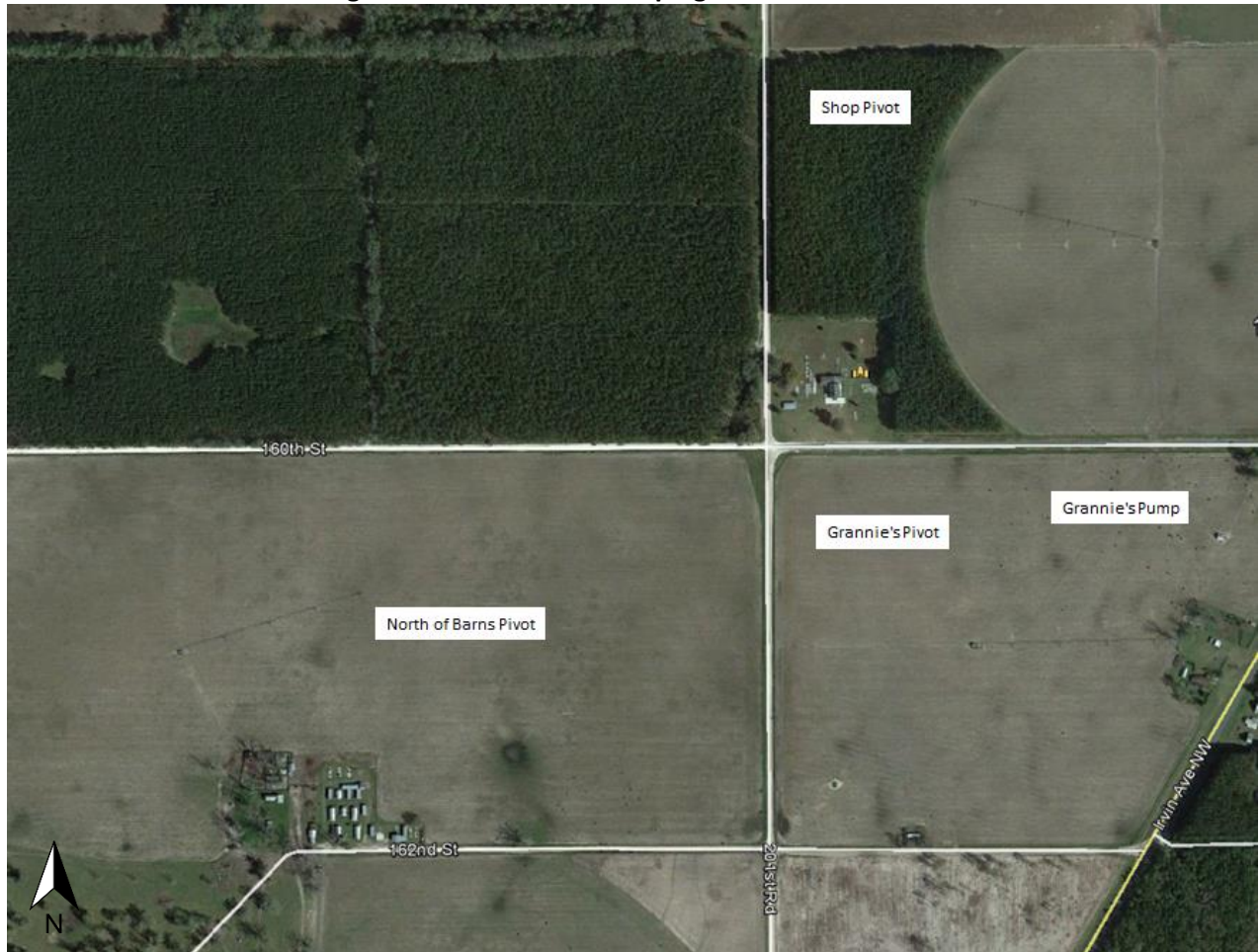
Figure AV.1. Grannie's Pumping Plant Aerial View
