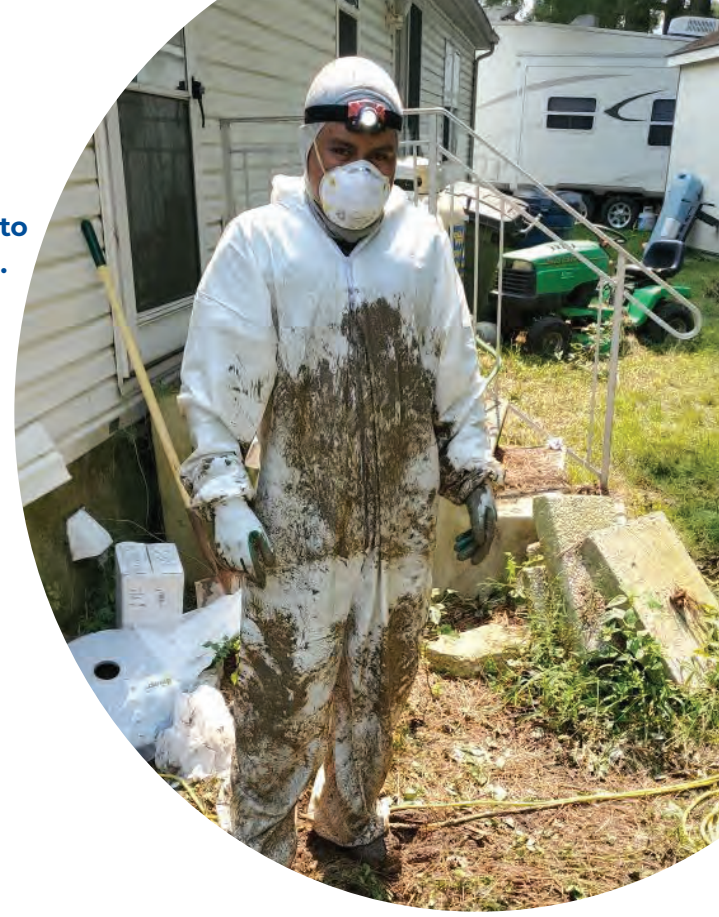
Contractor replacing a sump pump is a dirty job
